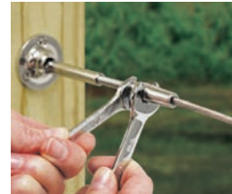
Tighten cone onto receiver.
