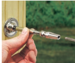
Fully seat wire rope.
