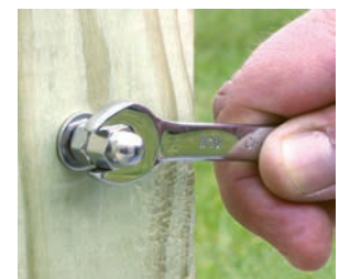
Step 3 Install acorn nut
