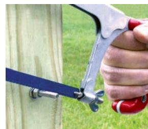
Step 2 Cut thread leaving 1/4”
